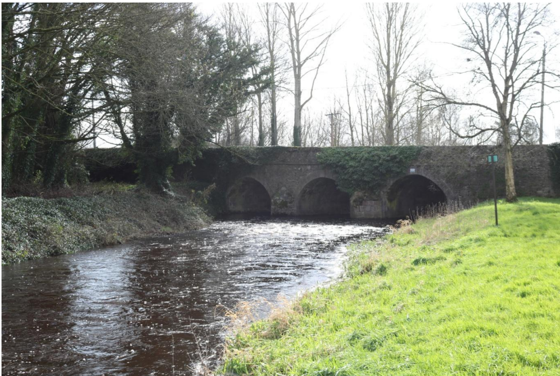
Figure 15: Proposed Development Area, Eighteenth century road bridge (NLAH 11810003) over River Slate, from east
