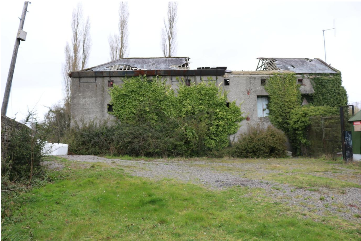
Figure 14: Malthouse (NLAH 11810038) from south
