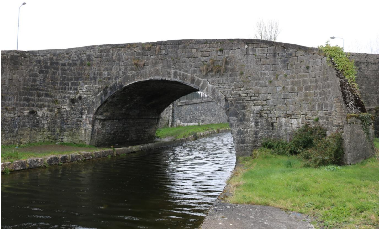
Figure 12: Bridge (NLAH11810015) over Grand Canal, from west
