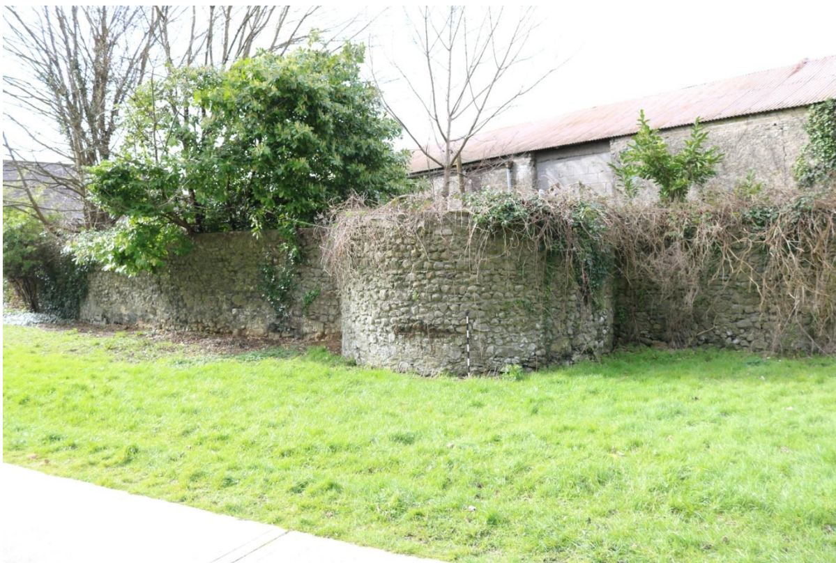
Figure 18: Bowed projection from rubble-stone wall (NLAH 1810004) parallel with Slate river, from east
