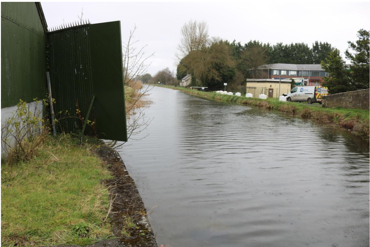
Figure 13: Grand Canal (Athy Branch) tonpath from east
